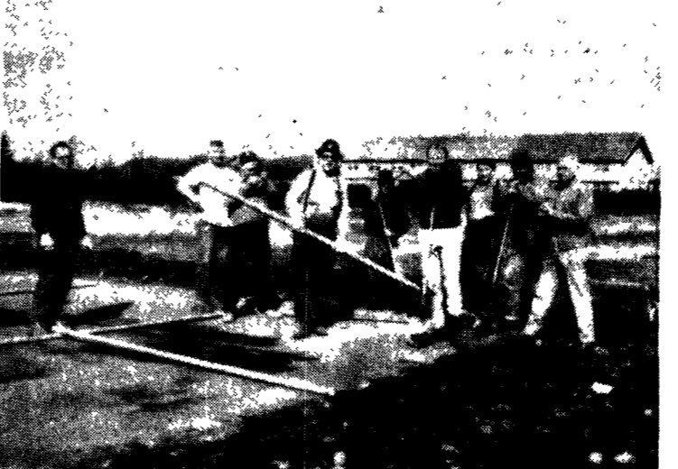
Last Saturday the Lions Club of Forks held a work party at Tillicum Park to erect a new fence around the tennis courts. A good sized group showed up under partly sunny skies to get things started, and the gentlemen were able to, by the end of the day, get all the fence posts and cement laid. They are now waiting to receive more fencing to complete the job, which they hope will be in another 2 weeks. Happy tennis playing, thanks to the Forks Lions Club.
